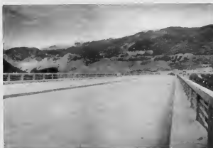
This view shows the finished surface of Bridge No. 1. Whereas the old road from Catia to the sea didn't have bridges, the new highway makes use of modern spans such as shown to facilitate comfortable, safe travel.
